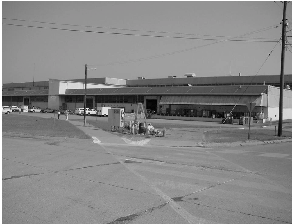
Figure 1.2 C-720 Maintenance Shop at the PGDP
